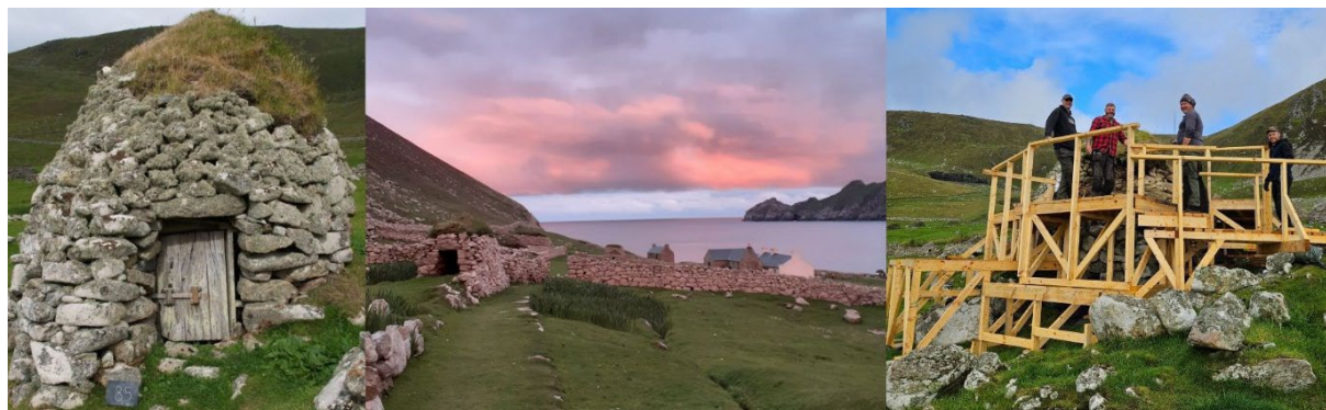
Images L-R: Repaired cleit on Hirta; summer sunset St Kilda; cleit repairs in action, Hirta (© National Trust for Scotland)
