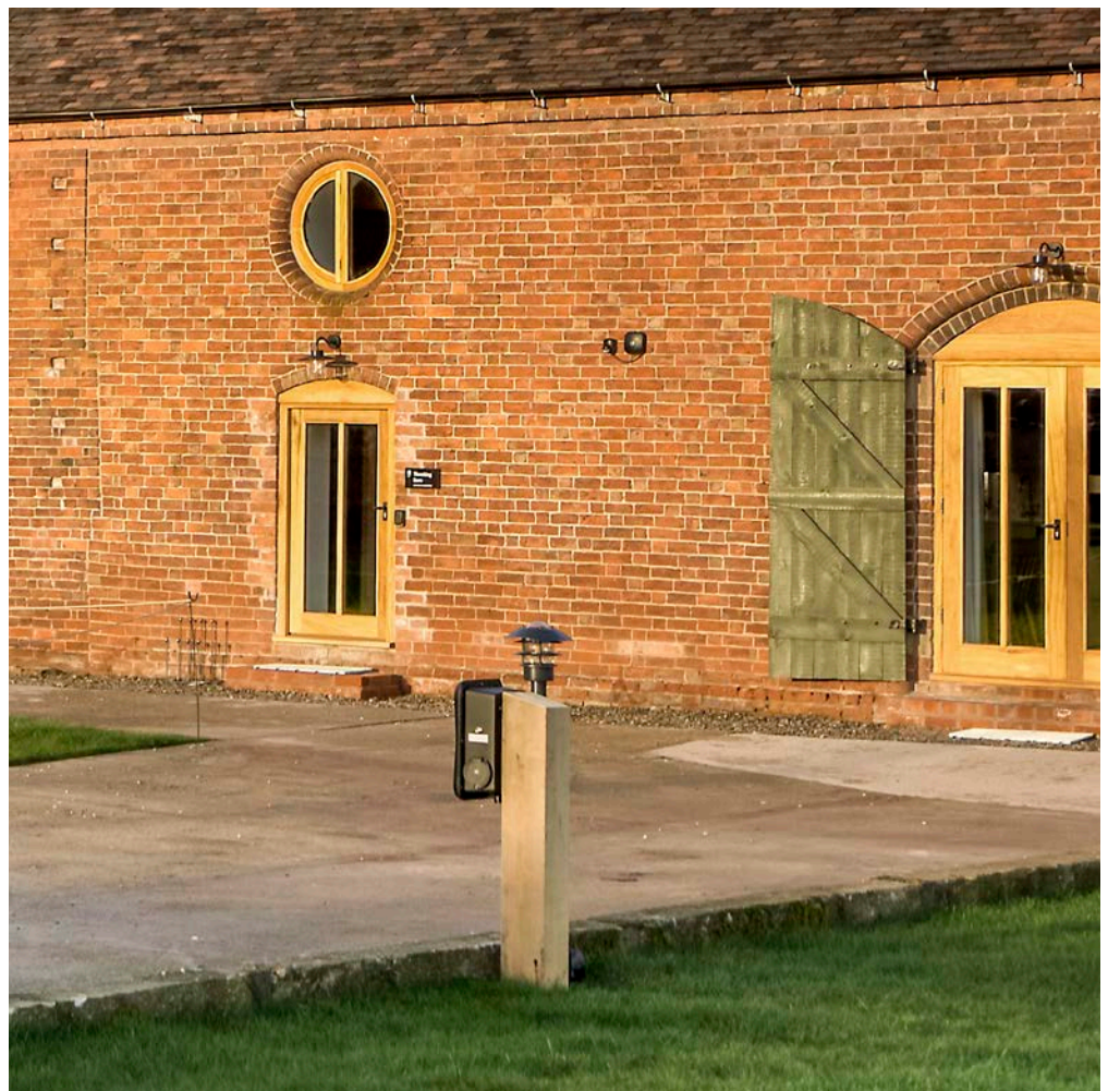
Figure 13: At this barn conversion, a freestanding electric vehicle charging point is attached to an external light. © National Trust
