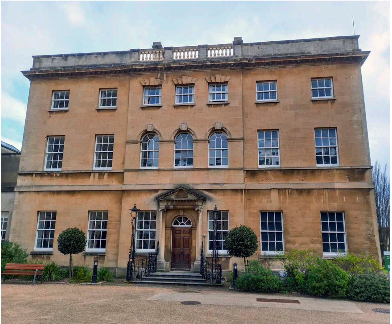
Figure 11: Air source heat pumps have been installed in an inconspicuous location to the right-hand side of the door and are barely visible on the front elevation of the Grade I listed building.
